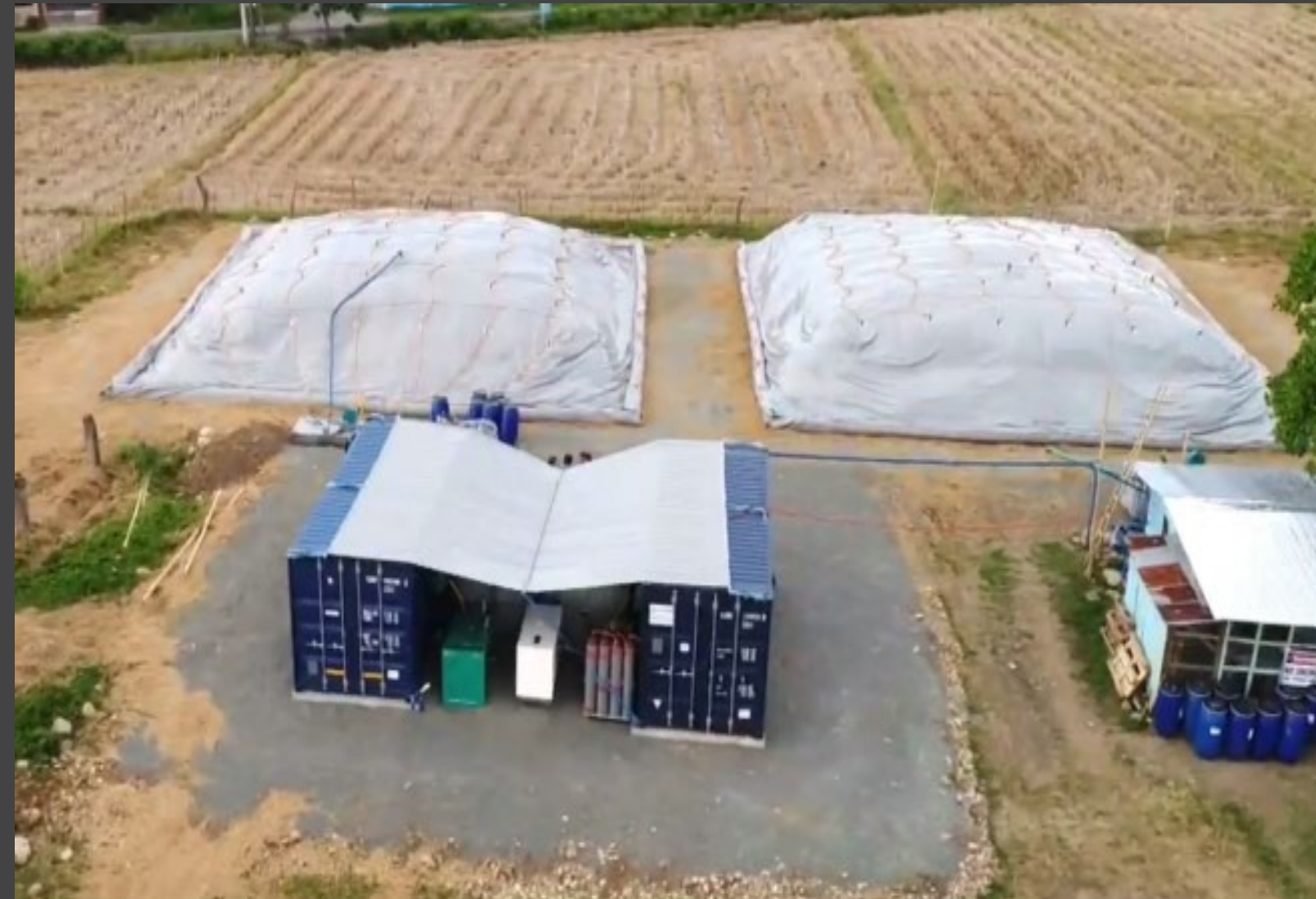
Rice Straw Biogas Facility in the Philippines (Straw Innovations)
